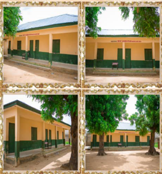
Construction of one block 3 Classrooms at Dr. Sayyadi Junior Secondary School, Ringim Town
