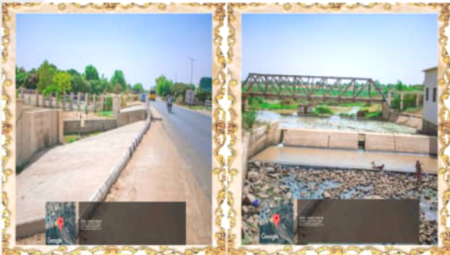
Repair and Reconstruction of Bridge at Gada, Kazaure LGA
