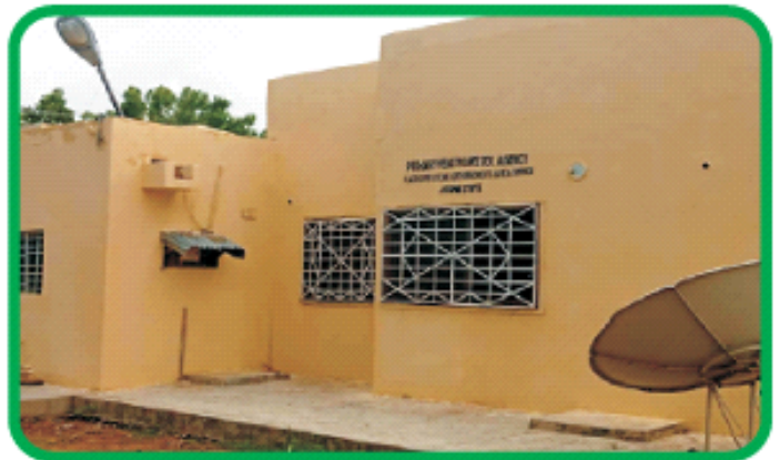
Renovated PHC Office, PHC Dunguyawa, PHC Katsinawa and corper's lodge
