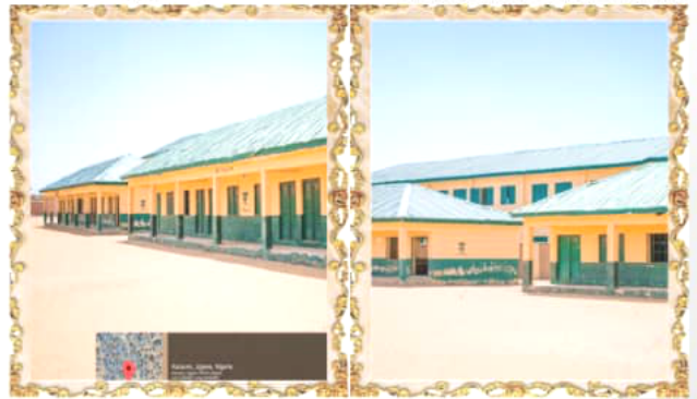
Provision of 2-Block 3 Classroom at Government Day Senior Secondary School, Kanti
