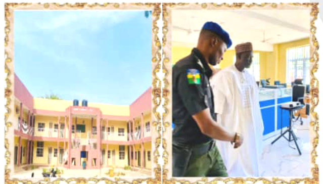
Construction Of Mathematics and Statistics Complex Hall at Hussaini Adamu Polytechnic College Kazaure
