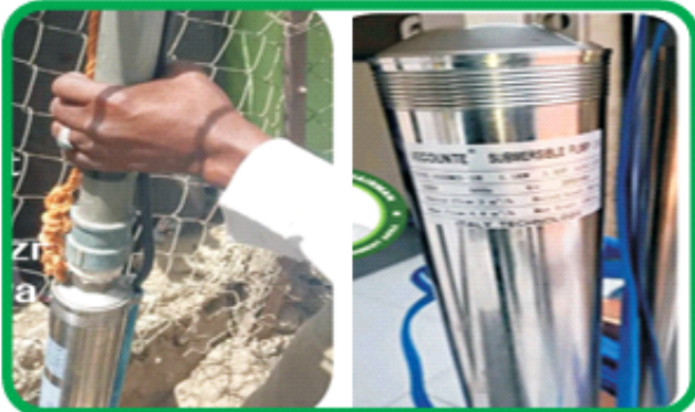
Installation of Solar & Electric submersible pumps at Galadanchi, Kafin Chiroma, Gallu, Sabaru, Dunguyawa and Babbar kuka Kazaure
