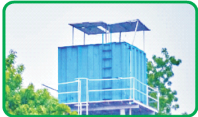
Repairs of (24) water supply points in various communities
