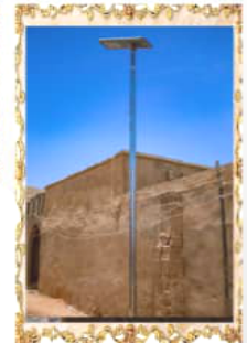
Installation of 200 no. 3-in-1 Solar Street Lights
