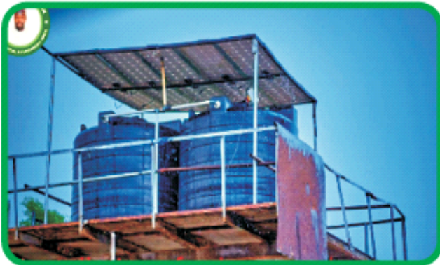
Conversion of existing boreholes to Solar power system in selected area eg Layin Abba Gurgu, Masallacin Idi etc.
