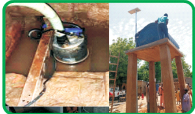
Installation of electric surmisable pump at Babbar Kuka behind Local Govt. Secretariat & Drilling and installation of Solar overhead tank at Kyankyaro & Tsedau town
